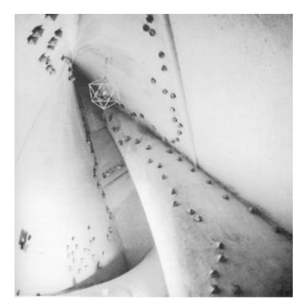
FIGURE 8.3 View, looking upward, of the inside of the Philips Pavilion. The objects on the surfaces are high-frequency loudspeakers in clusters, the patterns designed by Xenakis. Low-frequency loudspeakers were installed on the ground. From Treib (1996).
